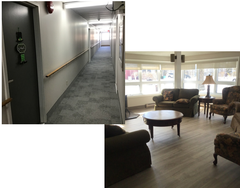
New Flooring Grant Grand Bend Non Profit Housing Corporation
